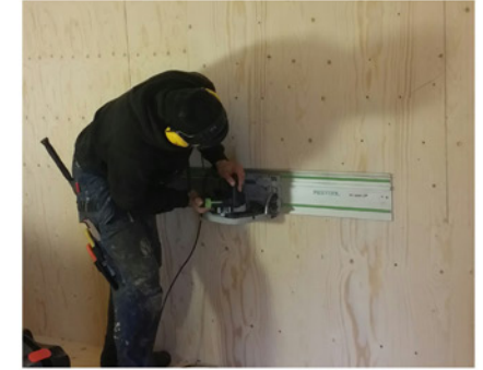
constructing the openings
