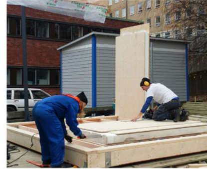
mounting the walls, screwing the elements to the slab
