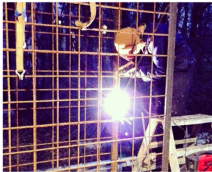
welding the gable
